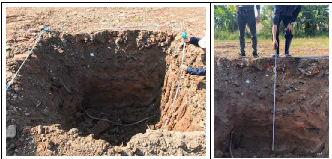
Fig. 3. Example of excavated pit for waste composition survey.
